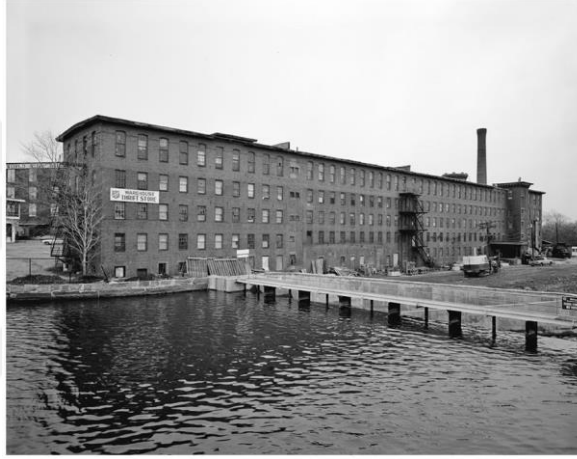
Şekil 4.2.1: Waltham, Massachusetts' Boston Manufacturing Co. Binası, Moody Sokağı'ndan görünüşü, Historic American Engineering Record, MA-54-5; HAER MASS, 9-WALTH, 4-5, Steve Dunwell, 1979, (Berens, 2010)
